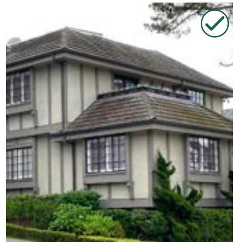
Stucco that is stained or painted and is either smooth or lightly textured is appropriate.
