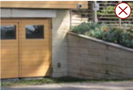
Large exposed retaining wall
