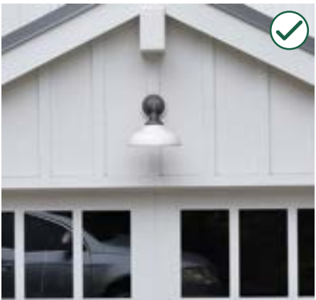
Locate and shield fixtures to avoid glare.
