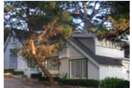
Varied roof lines
